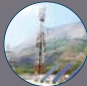
Amrita Wind Energy Centre
