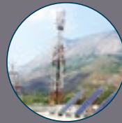
Amrita Wind Energy Centre
